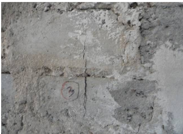
Fig. 5: Failure mode of modified rat-trap bond masonry under cyclic loading
